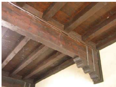
Double-frame floor viewed from below: the main beams can be seen with the secondary joists laid transversely.
